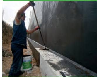
External basement wall
