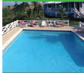
Swimming pool waterproofing
